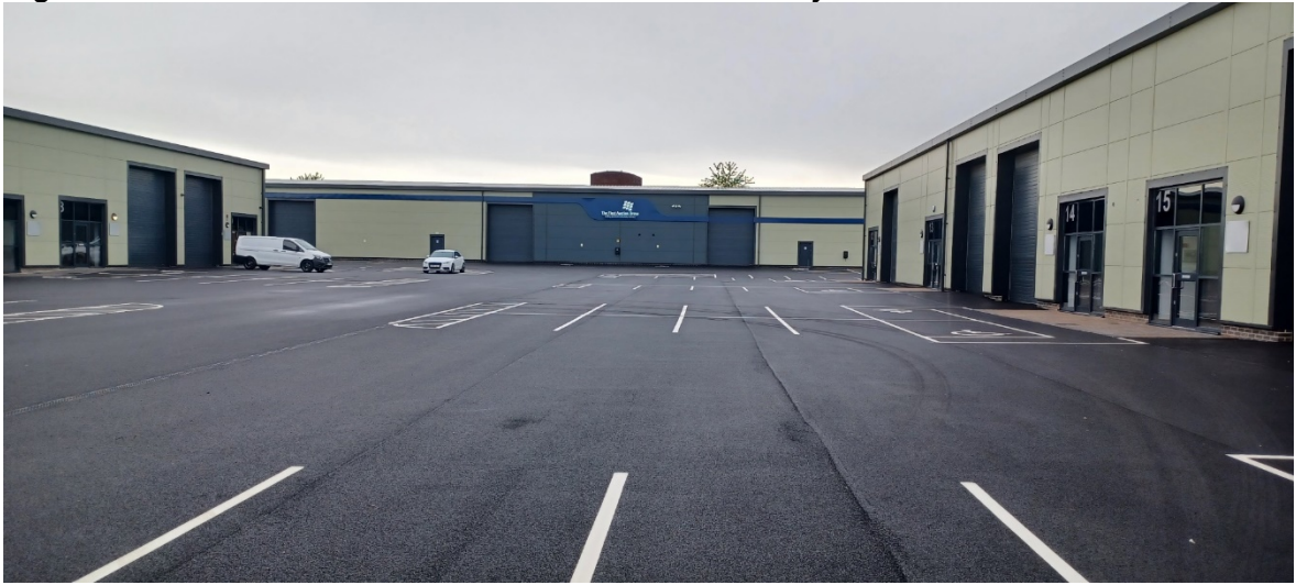
Figure 2 - Photo on site of P/20/1515/2 taken 9 th May 2023
